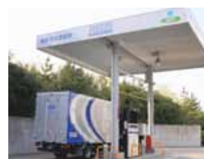
Private natural gas refueling station
